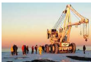
Modified cranes for heavy lifting
