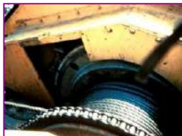
Loose or missing hardware, nuts, or bolts
