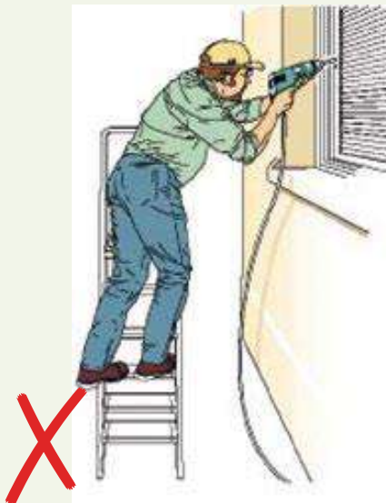
Incorrect – steps are side-on to work activity.
