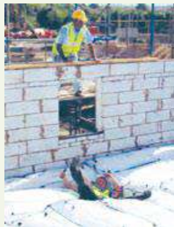
A worker falls into a soft landing system.
