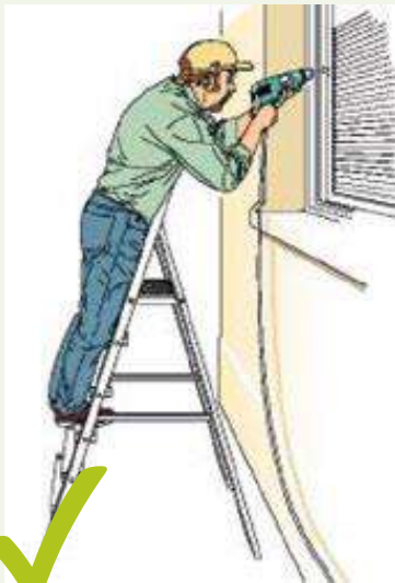
Correct – steps facing work activity.
