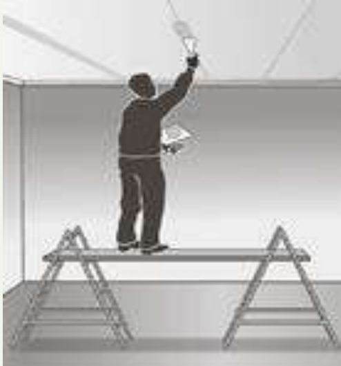
A worker stands on a trestle scaffold.
