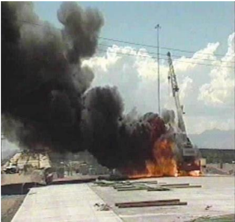
Crane in salt lake city explodes in flames when it touches a power line.
