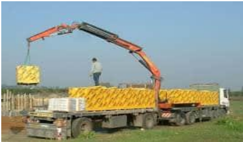
Lorry middle Loading Mobile Crane
